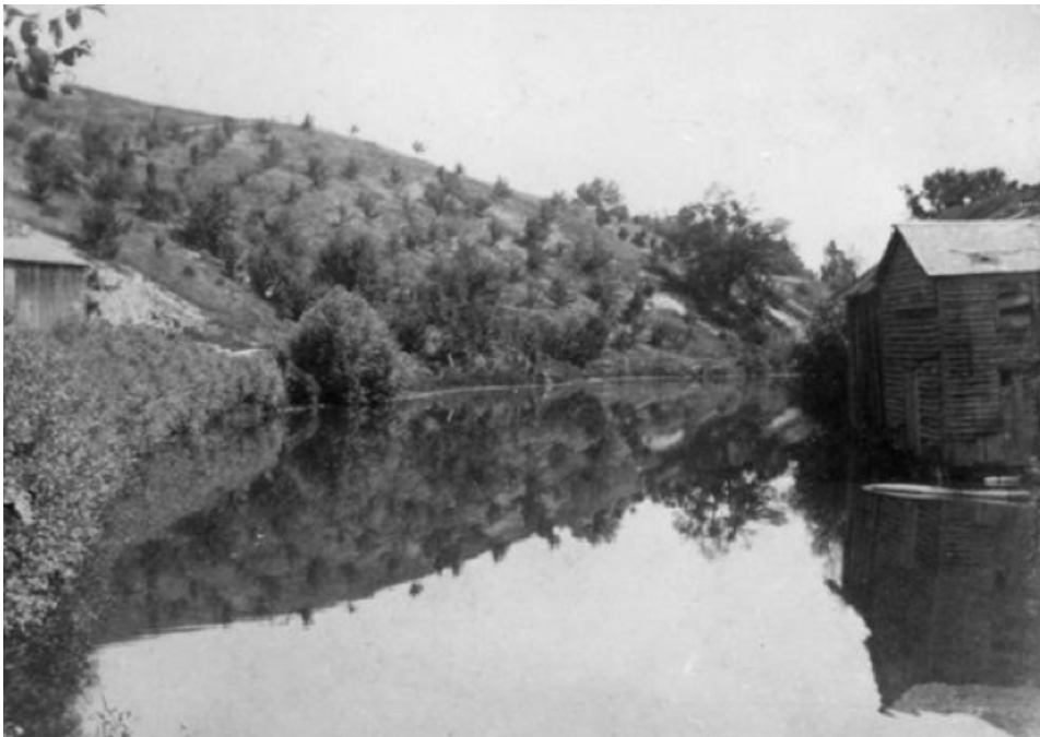
189. Historic view looking east from the Queen Street bridge, date unknown. (Source: courtesy of PAMA)
