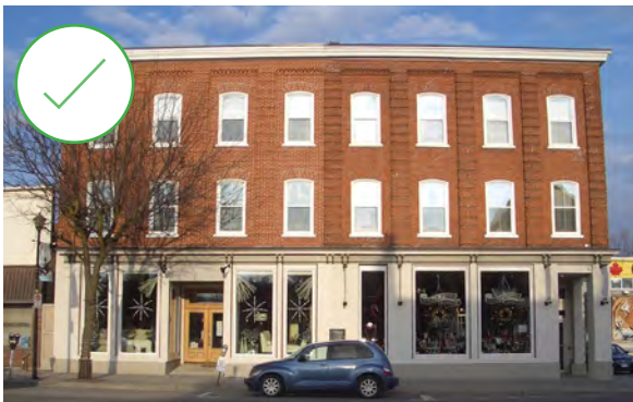
120. Left hand side of building was re-built following fire damage, Picton Main Street HCD. (Source: ERA)
