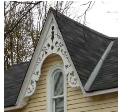
48. Maintain existing features such as this decorative bargeboard at 122 King Street East. This may require periodic repainting or refinishing. (Source: ERA)
