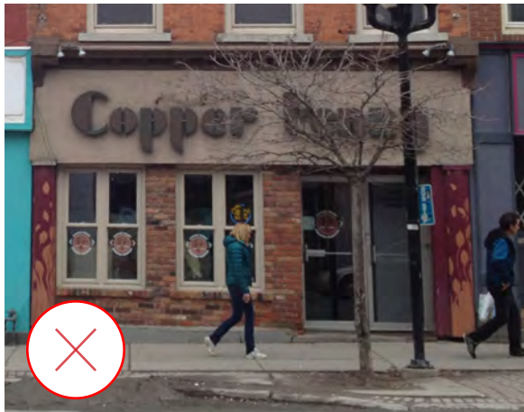
107. New storefront on a historic building that does not take into consideration the traditional components of a storefront or the proportions and architecture of the existing building, Kingston, Ontario. (Source: ERA)
