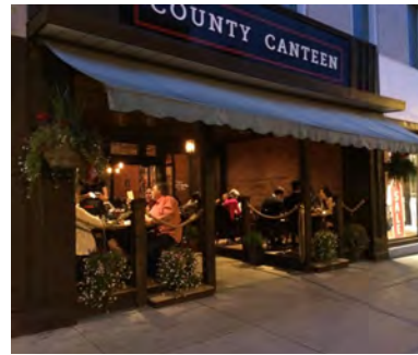
155. Recessed storefront with outdoor seating, Picton Main Street HCD. (Source: ERA)
