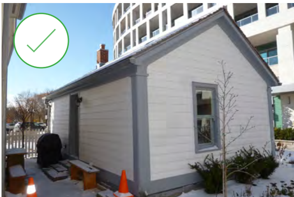
46. Hardie Board was used to repair one wall of this wood clad building in Bronte, Ontario. (Source: ERA)
