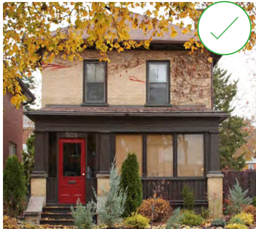
78. The enclosure of this historic porch maintains existing horizontal and vertical rhythms as well as architectural elements of this Edwardian Classical house in Peterborough, Ontario. (Source: ERA)
