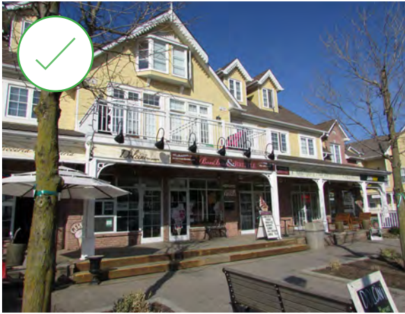
131. New mixed use development in Kleinburg-Nashville HCD with a house form design. (Source: ERA)
