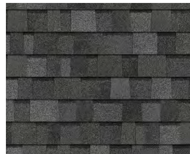
70. 3-tab asphalt shingle roofing. (Source: Roofpedia)
