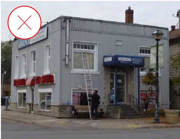
100. Original architectural detailing is concealed by modern metal cladding on 40 Queen Street North. In contrast to parging or stucco, this cladding could be more easily removed to reveal original cladding, design and detailing. (Source: ERA)
