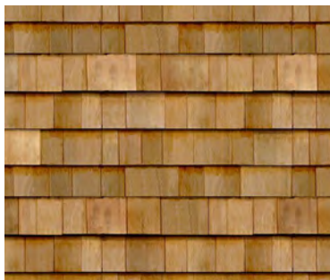
69. Wood shingle roofing. (Source: Nichololas Evanoff Roofing)
