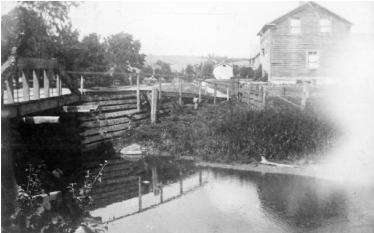
166. Humber River bridge at King Street East, date unknown. (Source: courtesy of PAMA)
