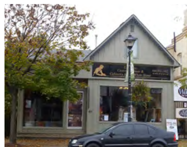
126. Pitched roof at 46 Queen Street North, Bolton. (Source: ERA)
