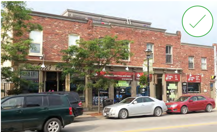
116. Note the location of signage within fascia board and external goose neck lighting on 52 Queen Street North as well as rooftop addition set back from front façade and largely shielded by parapet on 54-56 Queen Street North, Bolton. (Source: ERA)
