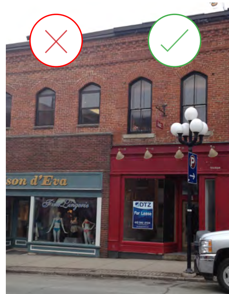
103. Note the difference between conserved historic windows on the right and the modern replacements on the left. The new storefront on the left does not take into consideration the original window glazing pattern and proportions and as a result the new windows are not compatible with the architectural style of the building, Kingston, Ontario. (Source: ERA)
