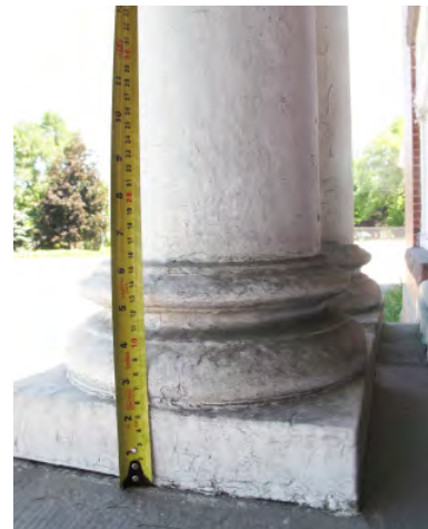
49. Investigate and document existing architectural elements prior to repair and restoration. (Source: ERA)
