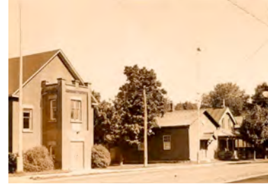
26. Town Hall and Orange Hall on King Street East. Date unknown, prior to 1940. (Source: courtesy of PAMA)
