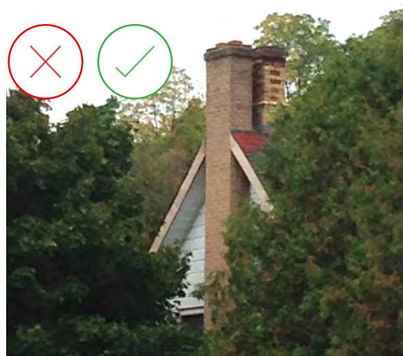
74. Retention of original chimney in contrast to installation of unsympathetic new chimney at 49 Queen Street South, Bolton. (Source: ERA)
