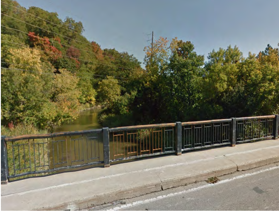
188. View looking east from the Queen Street bridge over Humber River. (Source: ERA)
