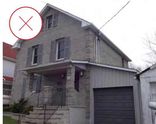
45. Grey brick cladding conceals original masonry and architectural detailing on this historic house in Kingston, Ontario (Source: ERA) (Source: ERA)
