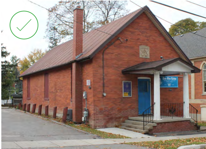
68. Appropriate use of metal roofing on gable roof at 16 Nancy Street, Bolton. (Source: ERA)
