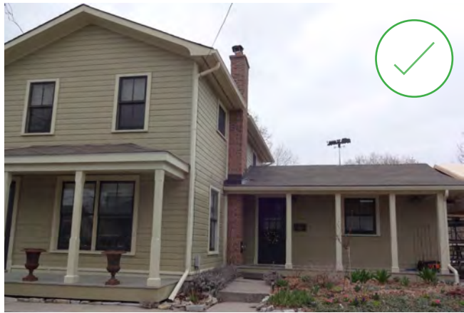
76. Compatible new porches on both principal house and addition, Barriefield HCD, Kingston, Ontario. (Source: ERA)
