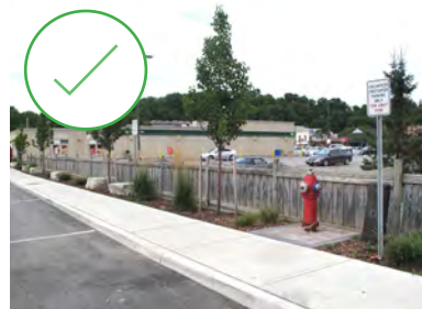
140. New landscaping that screens parking lot between Queen Street North and Ann Street, Bolton. (Source: ERA)
