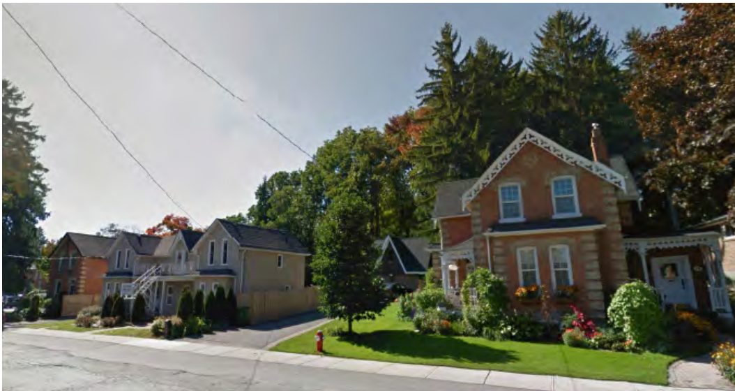
147. Temperance Street streetscape, Bolton. (Source: Google)
