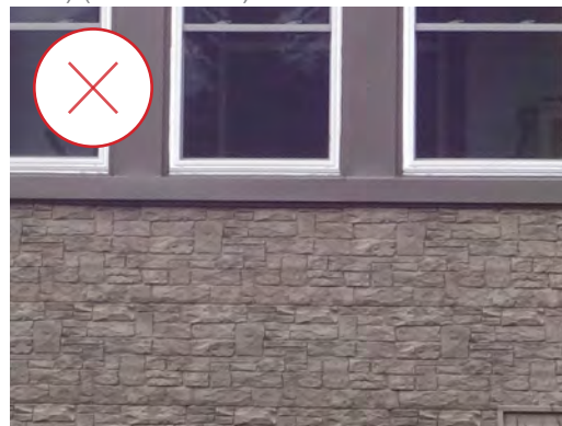
47. Artificial stone (seen here) or real stone cladding is not an appropriate material to use in Bolton. (Source: ERA)
