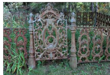
41. Plummer Foundry cemetery fencing, Mount Pleasant Cemetery, 16381 Mount Pleasant Road, Caledon. (Source: Town of Caledon)
