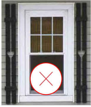
64. Inappropriately proportioned new shutters. (Source: www.oldhouseguy.com)
