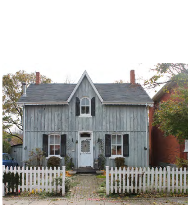
38. Wood picket fencing at 52 Sterne Street, Bolton. (Source: ERA)
