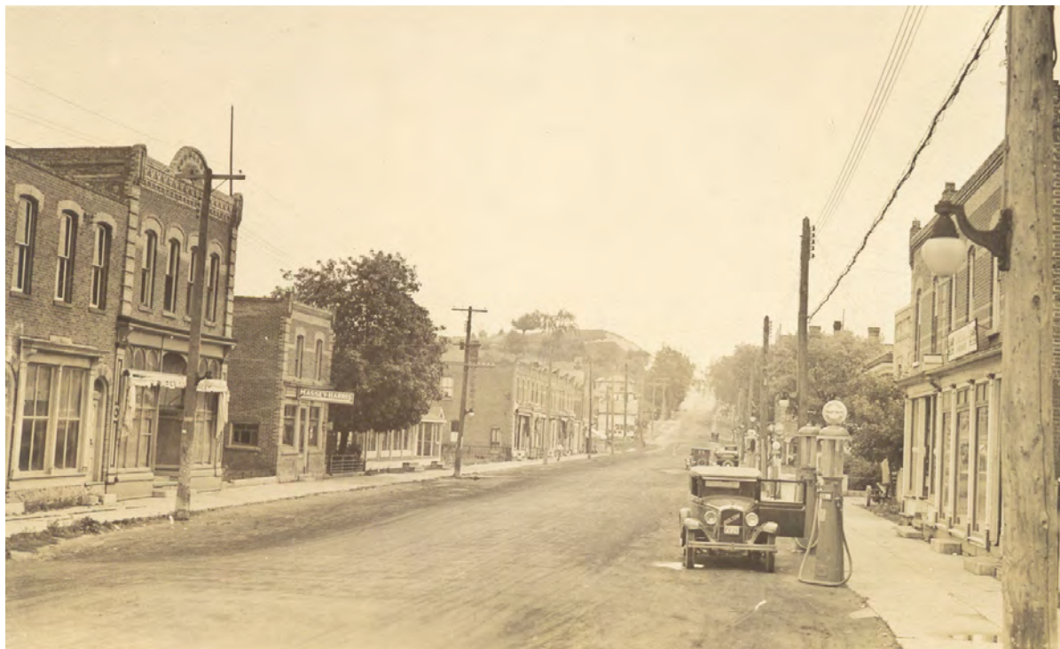
24. Bolton postcard c. 1920s, looking south on Queen Street. (Source: Town of Caledon)
