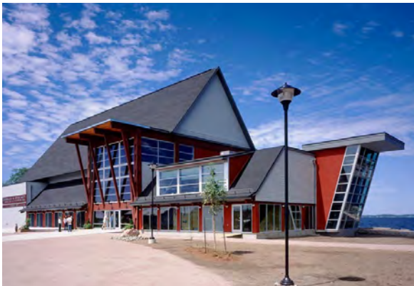
173. The Charles W. Stockey Centre for the Performing Arts is an excellent example of a multi purpose community centre. Designed to read as a ship, it is inspired by its setting and local historic narrative, Parry Sound, Ontario. (Source: Stockey Centre website)
