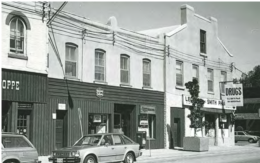
137. 1, 3, 5, 7 and 9 Queen Street North façades concealed by metal sheeting and stucco in the 1980s, Bolton. (Source: Town of Caledon)
