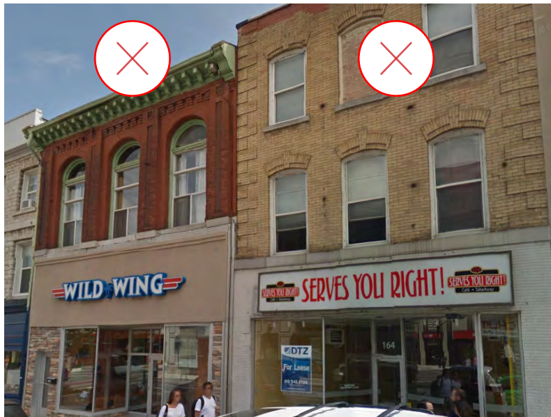
113. The signage on the left is inappropriately proportioned, obscuring architectural detailing on the historic building. The signage on the right is correctly located but the box design with internal lighting is not compatible with the architectural style of the building or the character of the streetscape, downtown Kingston. (Source: Google)
