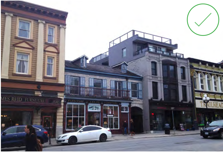
115. Rooftop addition on historic commercial building in downtown Kingston. The addition has a simple design and is set back from the front façade, which minimizes its impact on the historic building. (Source: ERA)
