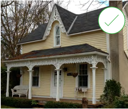
75. Well maintained historic porch, 122 King Street East, Bolton. (Source: ERA)
