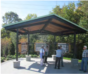
171. The new heritage interpretation pavilion at Humber River Heritage Park next to the Humber River Queen Street bridge, Bolton. (Source: ERA)
