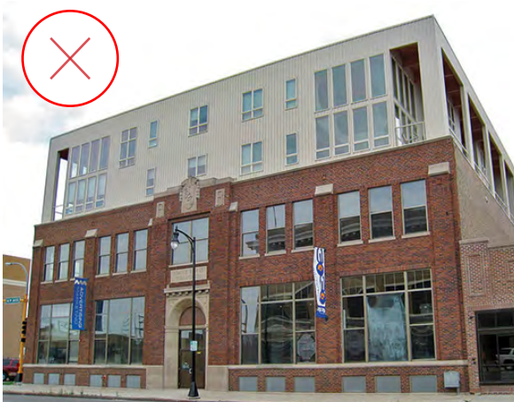
117. Rooftop addition that overwhelms the scale of the existing building. (Source: National Park Service, U.S.)
