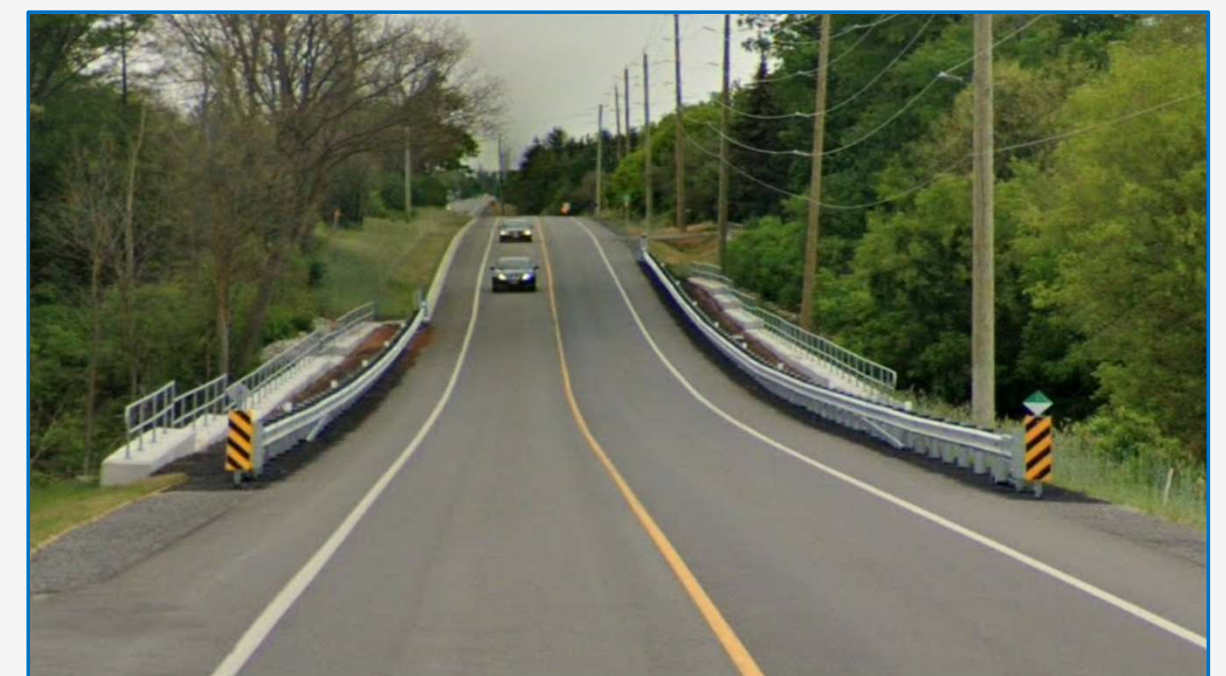
Typical road rehabilitation project example
