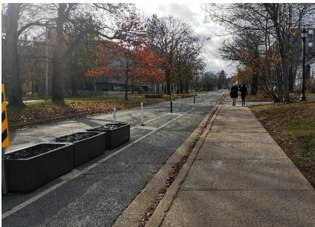
On-road protected bikeway with planters and flex posts (Halifax, NS)
