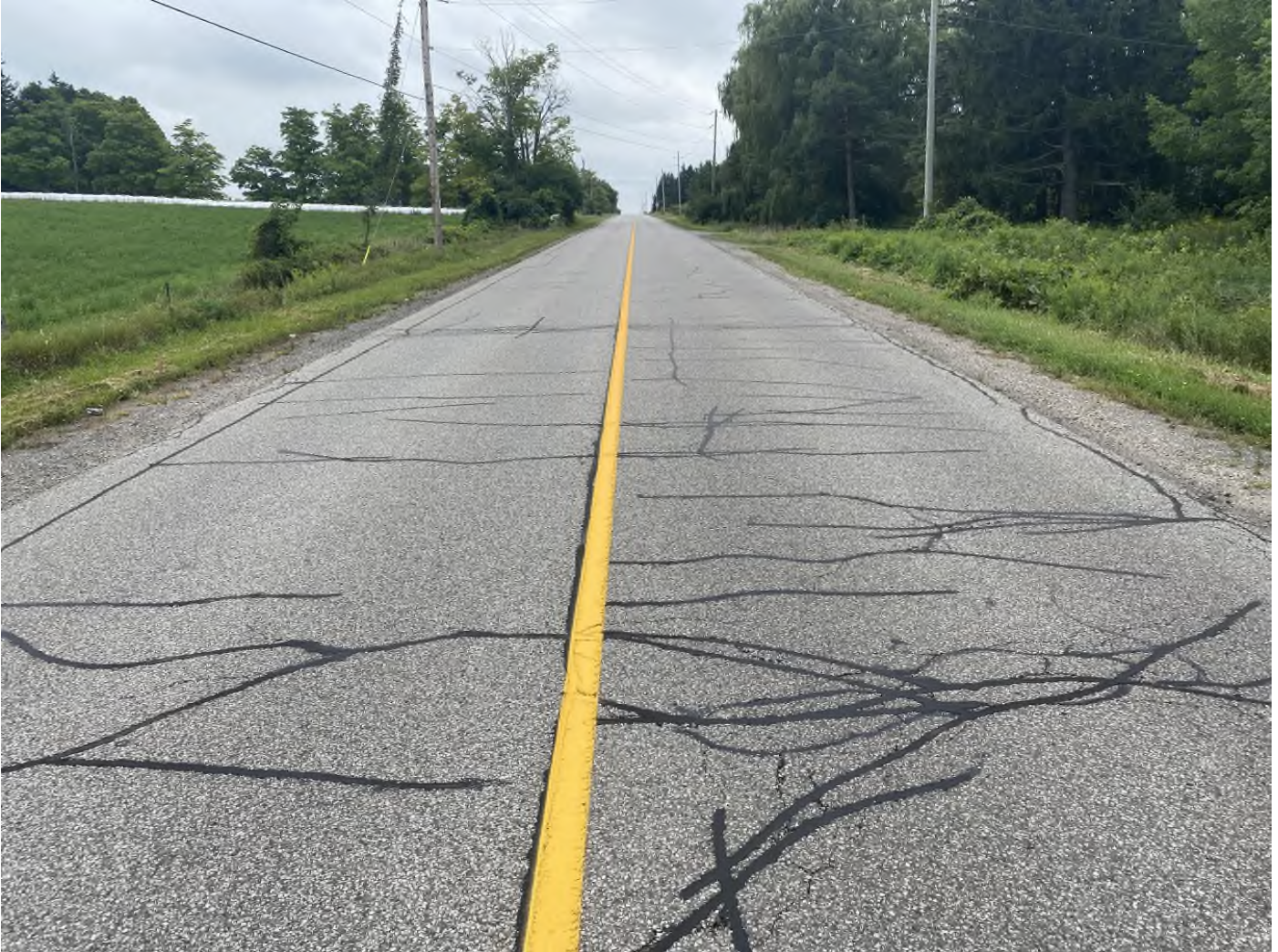
Rural Road Crack Sealing
