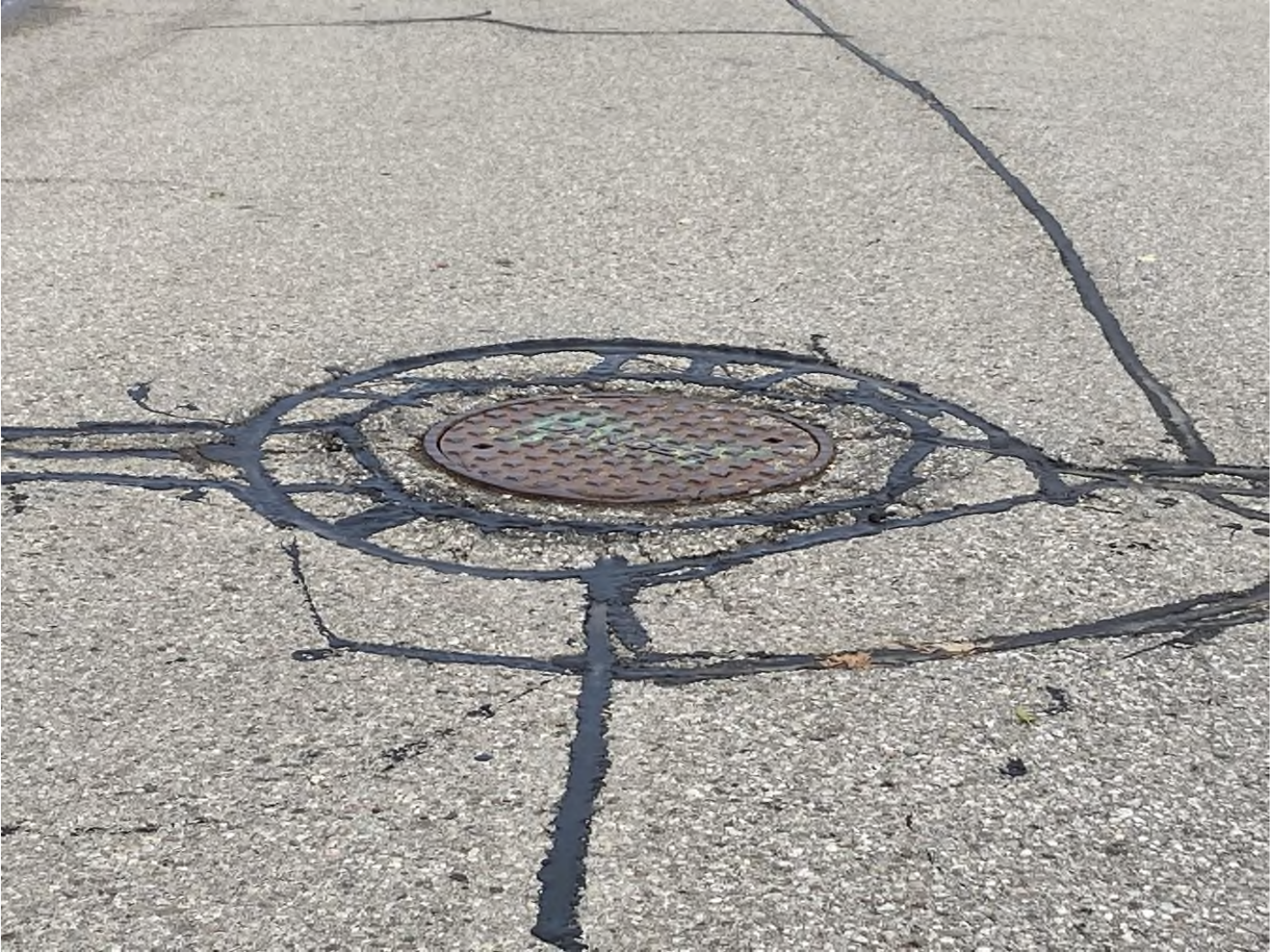
Crack Sealing End Result
