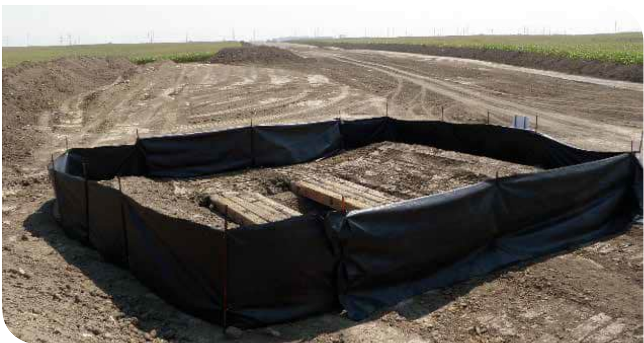
Cleaning station at construction site.
