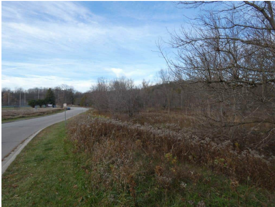
Photo 11: View northbound along the eastern shoulder of Deer Valley Drive. November 10, 2022.
