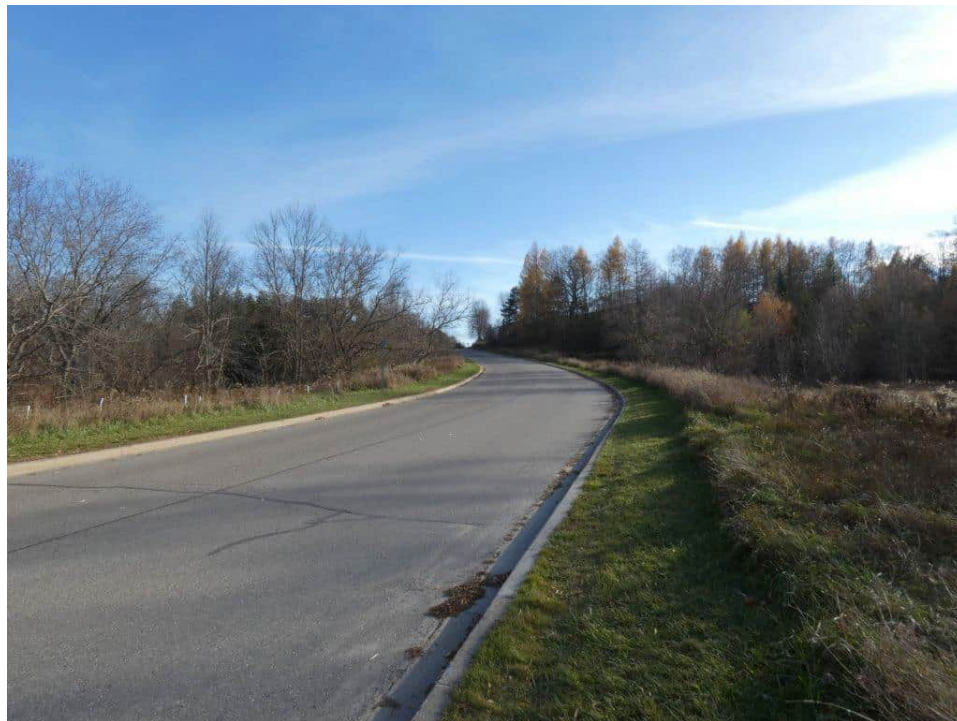
Photo 10: View southbound along the western shoulder of Deer Valley Drive. November 10, 2022.
