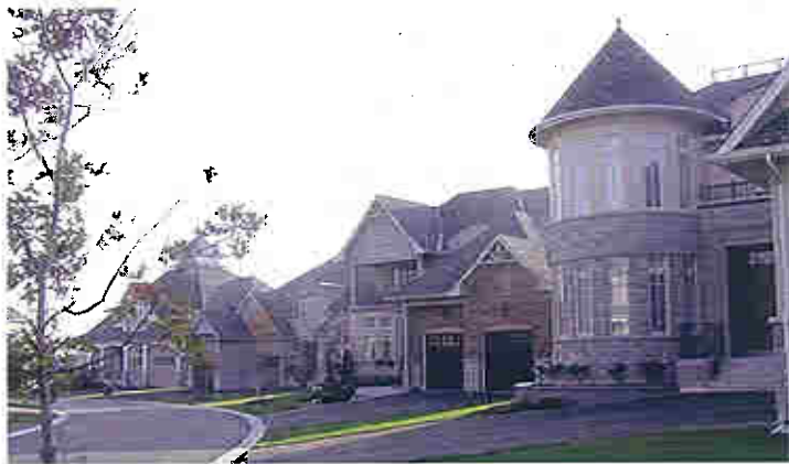
Building Projections Help to Visually Enhance the Streetscape
